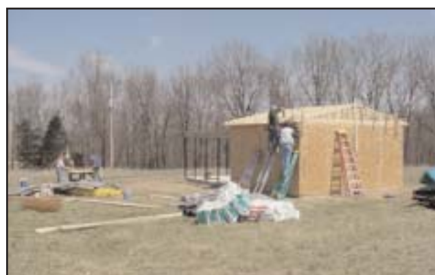
Members of the S.O.W.E.R.S. are busy building the observatory at NLR.
